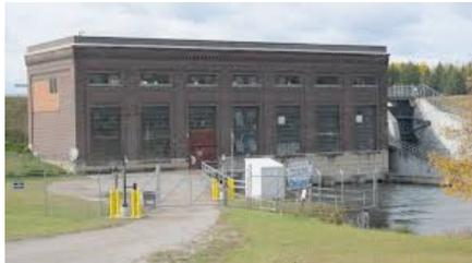
The Five Channels Dam is capable of producing 6,000 kilowatts, the hydro was completed in 1912. This hydro is named for the nearby location on the AuSable River where there were once five distinct river channels.
